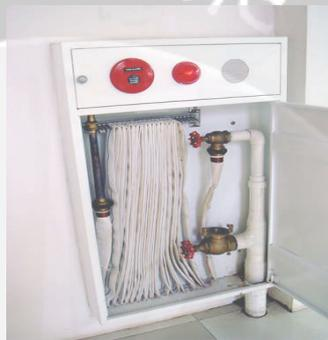
Gambar 3.19. Hydrant didalam Bangunan
