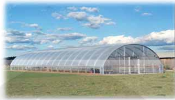
Gambar 2.13 Struktur Greenhouse Quonset.
