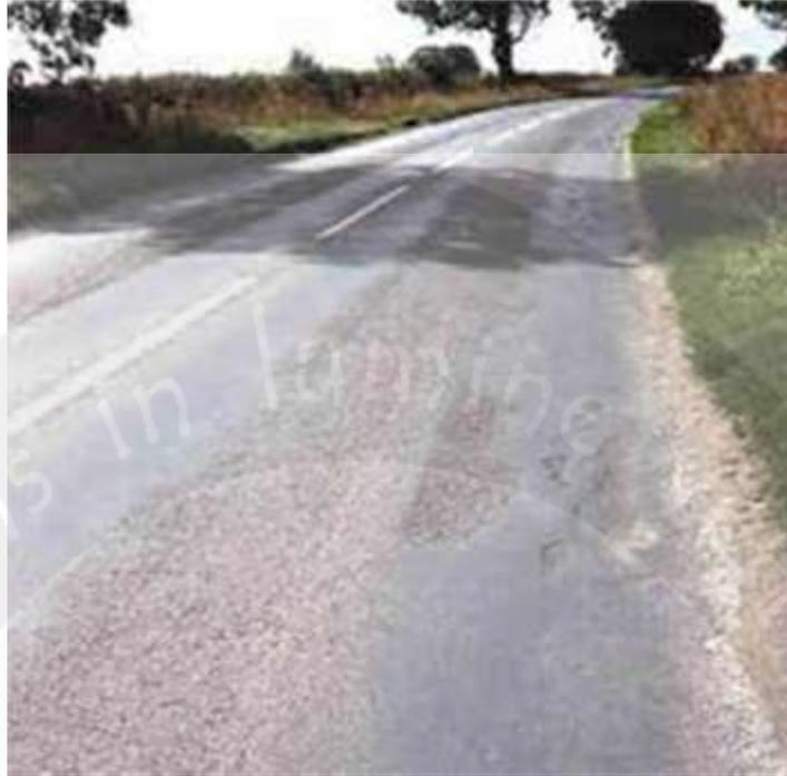
**Gambar 2.16** Pengausan (*Polished Aggregate*)
