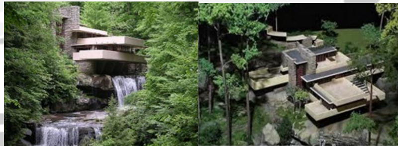
Gambar 3.5 Falling Water, Frank Lloyd Wright
