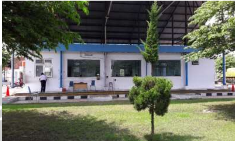
Gambar Lampiran 5-1 Jembatan Timbang Kalitirto
