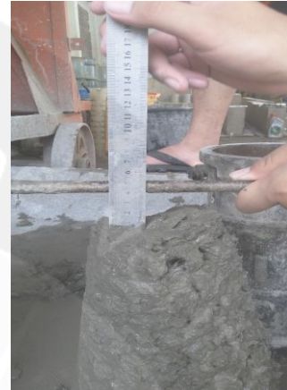
Nilai Slump Beton
