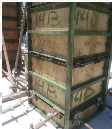
Fig. 2.2 Knock Down Formwork
