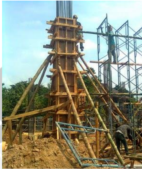
Fig. 2.1 Conventional Formwork
