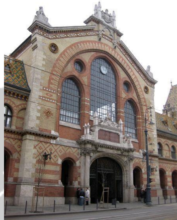
Gambar 2.24. Area Entrance Great Market Hall Budapest
