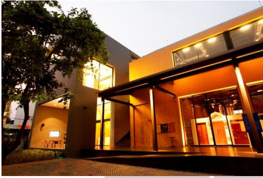
Gambar 2.6 Thailand Creative and Design Centre Sumber: http://www.archdaily.com/
