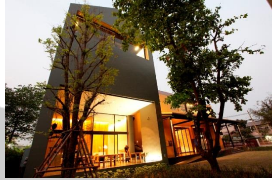
Gambar 2.7 Thailand Creative and Design Centre Sumber: http://www.archdaily.com/
