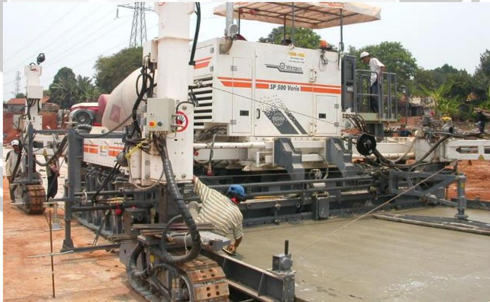
Gambar 2.1 Perkerjaan *rigid pavement (concrete paver)*
