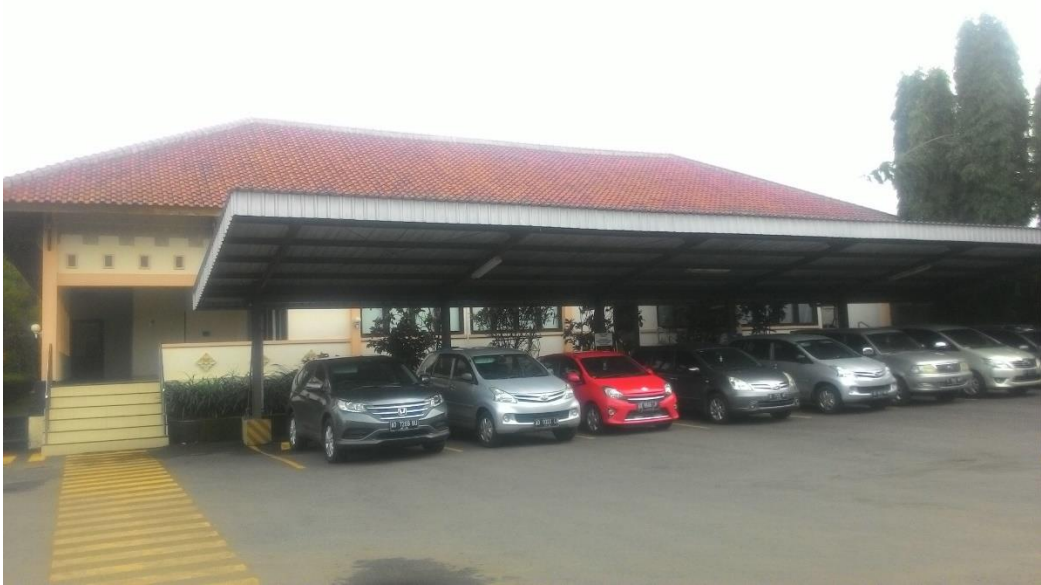
Gambar 4.3.4 – Lapangan parkir Office
