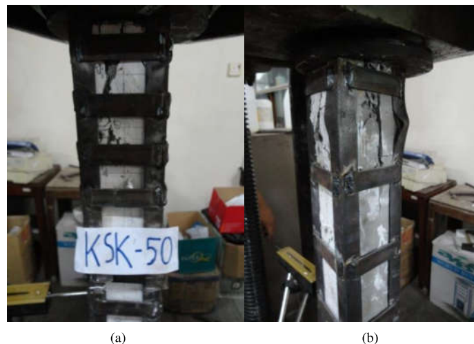
Fig. 4. (a) Crack propagation of concentrically loaded column; (b) Local buckling of angle steel shape of concentrically loaded column.
