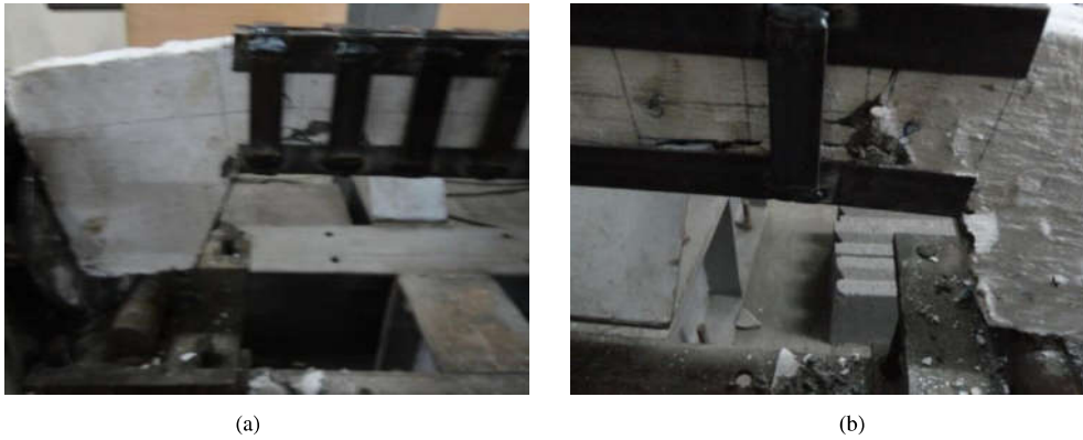
Fig. 6. (a) Crack pattern of the specimen KSV-50; (b) Crack pattern of the specimen KSV-150.
