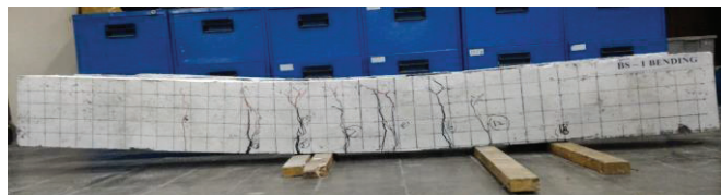
FIGURE 6. The crack pattern of BS1
