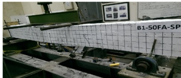
Fig. 5. The crack pattern of B1-50FA-SP specimen.
