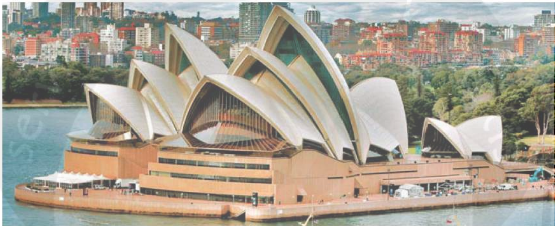
Gambar II.5 Gedung Sydney Opera House
