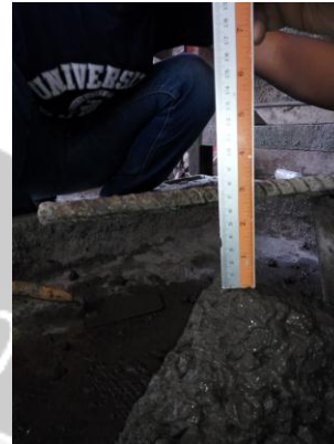
Proses Pengukuran Slump
