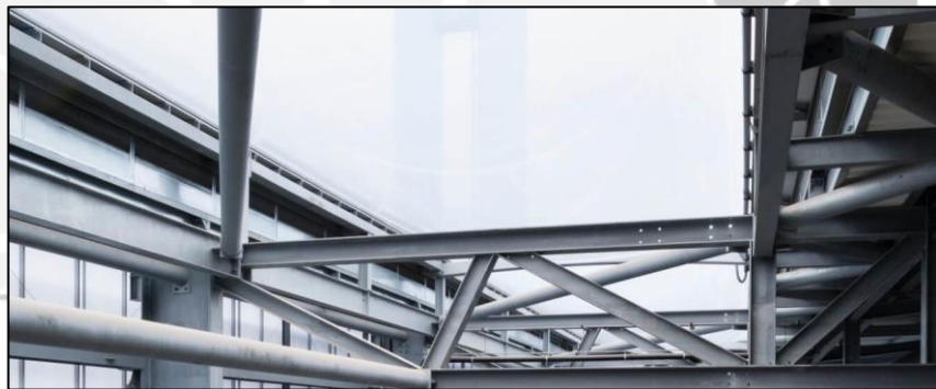
Gambar 2.24 Boiler room Suffolk energy-from-waste facility
