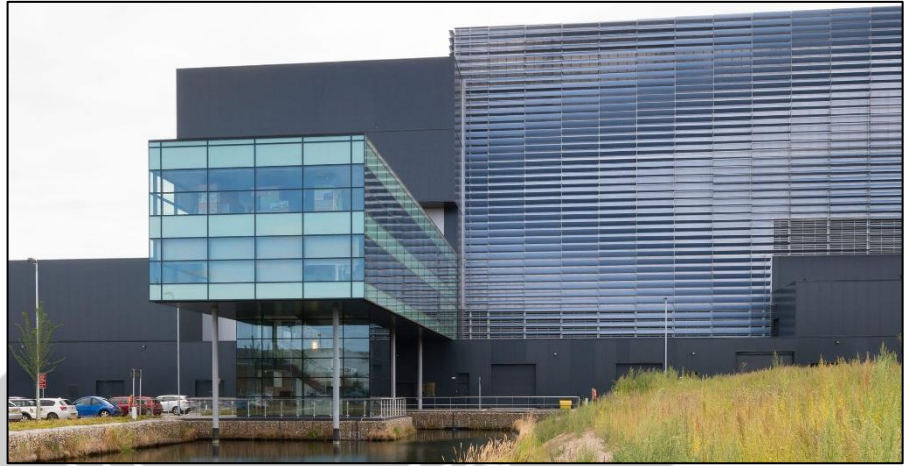
Gambar 2.17 Entrance Suffolk energy-from-waste facility
