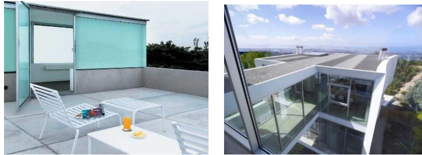
Gambar 5.57: Atap Dak Beton
