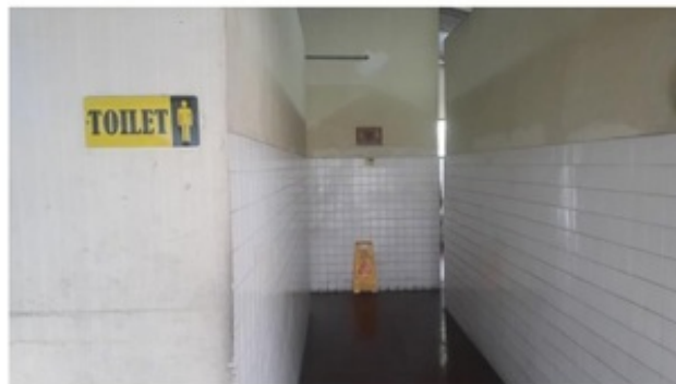
Figure 2.13 Toilet in PT. Kanisius
