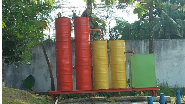
Figure 3.25. Wastewater Treatment Plant
