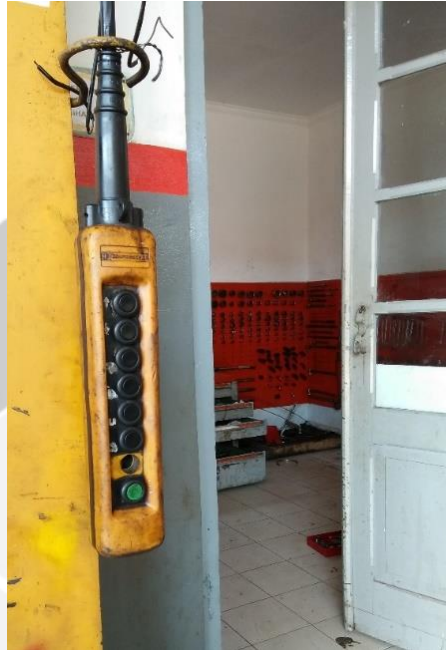
Figure 4.6. Crane placement in front of Tools Room
