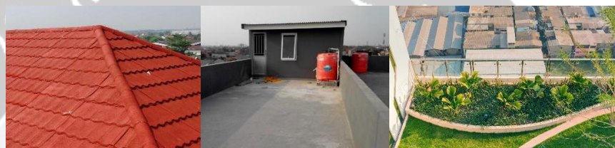
Gambar 6.9 : Atap Genteng Tanah Liat, Atap Dak Beton, Roof Garden
