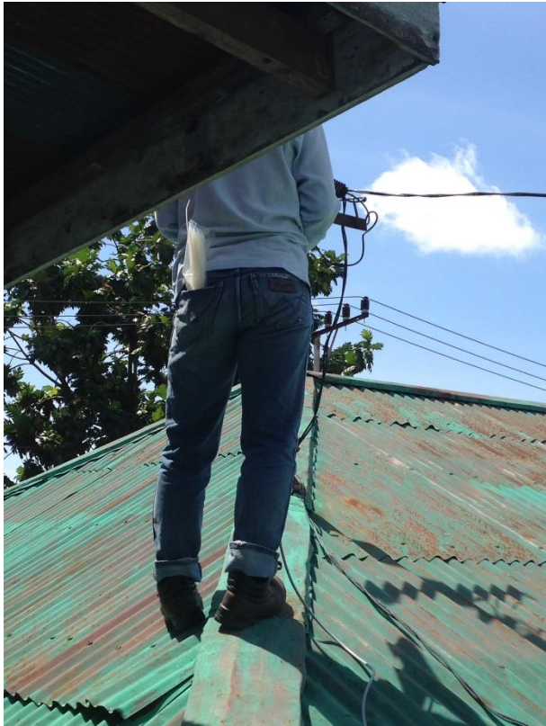
Gambar 14. Instalasi Radio Station (Residential)
