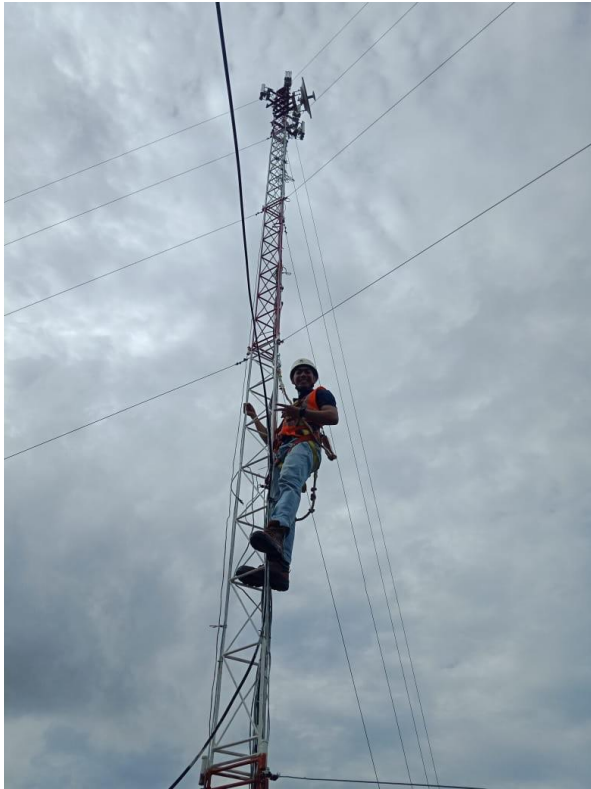
Gambar 8. Instalasi Radio Access Point
