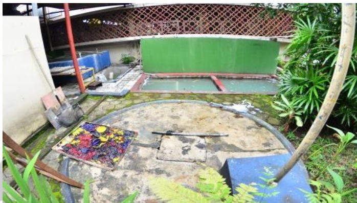
Figure 2.15. Liquid Waste Treatment Area
