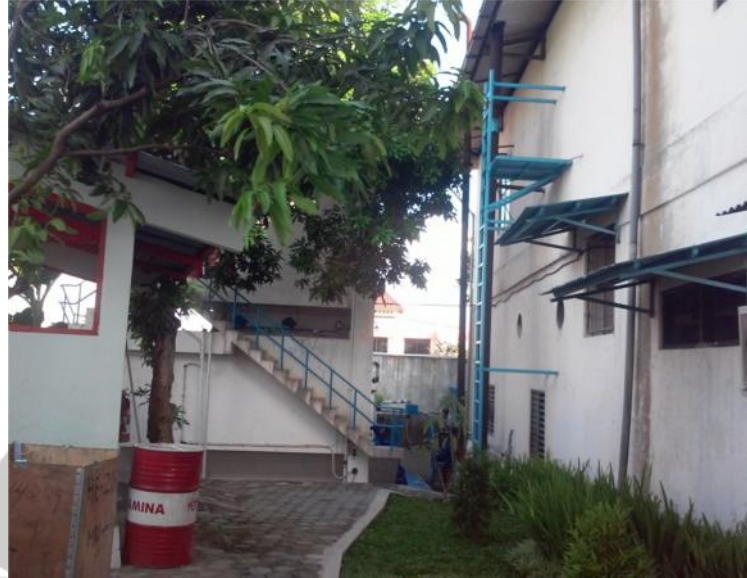
Gambar 2.8 Unit Pengolahan Limbah PT. Macanan Jaya Cemerlang
