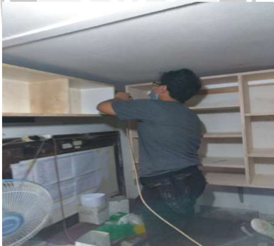
Picture 4.4. New Storage Installation
