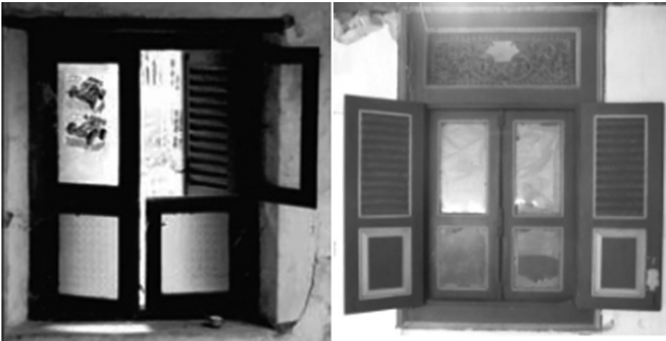
Figure 1. Various type of krepyak windows. Source: Kotagede Heritage District Yogyakarta. Homeowners' Conservation Manual (UNESCO, 2017).
