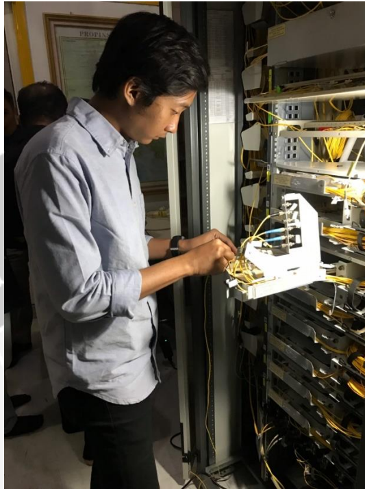
Gambar 5. Proses Pelabelan Kabel Di Optical Terminal Box
