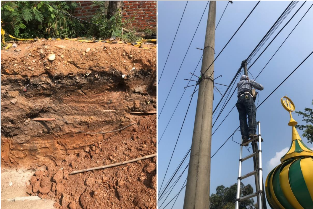
Gambar 3. Proses Penarikan Kabel Fiber Optic
