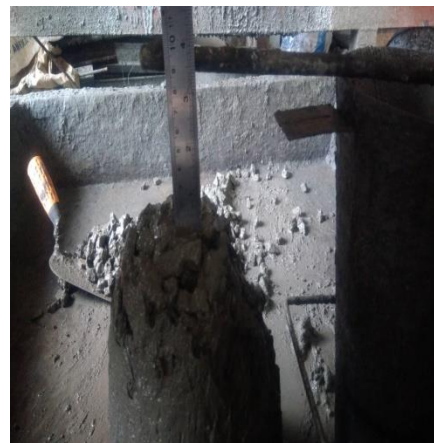
Proses Pengujian Slump
