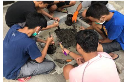
Proses mixing beton
