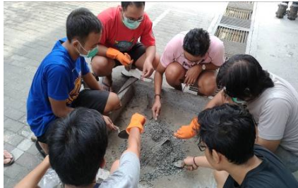
Proses mixing beton
