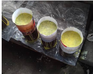
Proses caping beton
