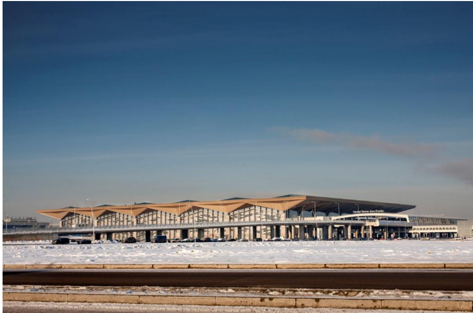
Gambar 2.29 Pulkovo International Airport Sumber: wikipedia.org, Pulkovo International Airport Architects: Grimshaw Architects, Ramboll, Pascall + Watson Location: Pulkovo VIP International, Pulkovo Airport (LED), Saint Petersburg, Russia, 196140 Project Year : 2014
