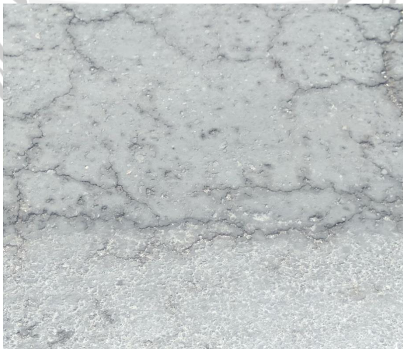
Lampiran C.8 Gambar Kerusakan Pengausan
