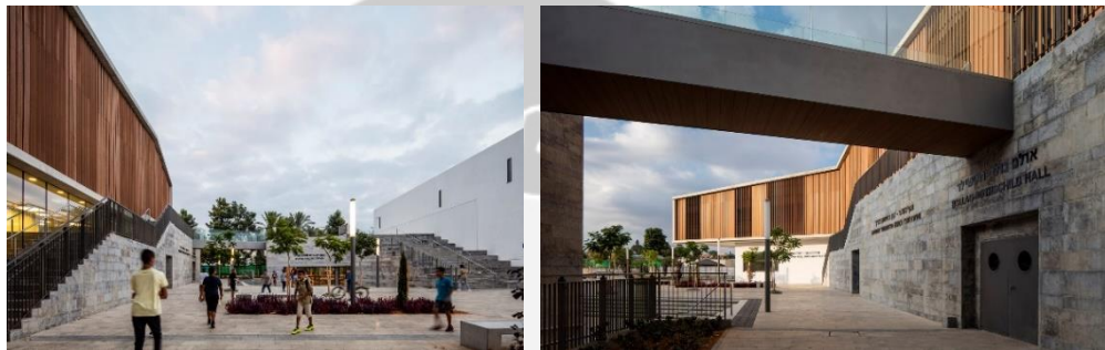
Gambar 2.10. Suasana Amphiteater dan Bridge Rehovot Community Center
