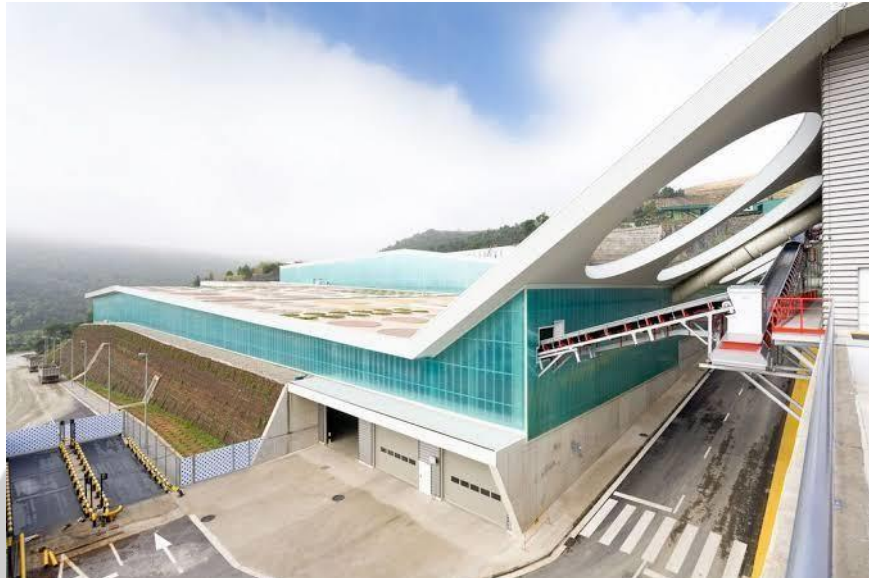
Gambar 2. 5 Waste Treatment Facility (Barcelona)
