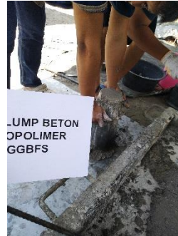
Proses Mixing Beton Geopolimer
