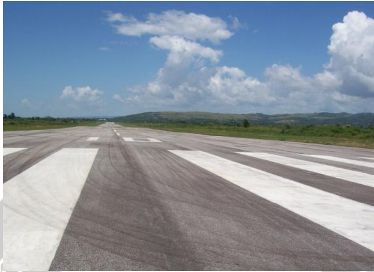
2. Run Way Bandara Tambolaka
