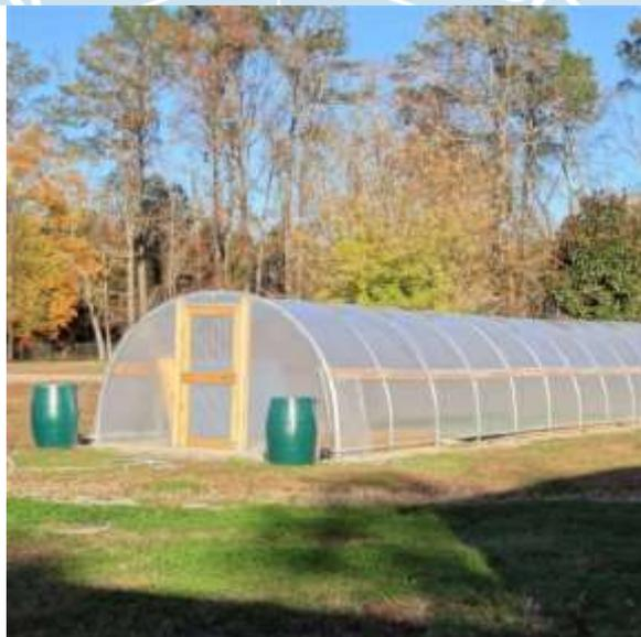
**Gambar 2.12. Tipe *Tunnel***
