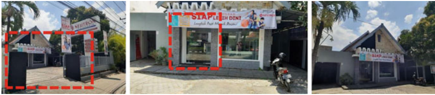
Fig. 3 The main entrance and parking area of neutron building
