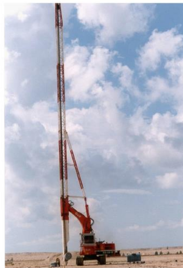
High power installation rig (Cofra b.v.)
