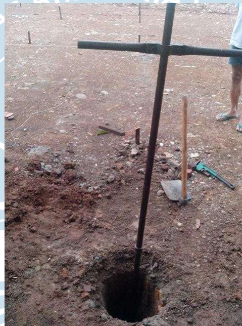
Gambar 3.9 Bored Pile Manual/Strauss Pile
