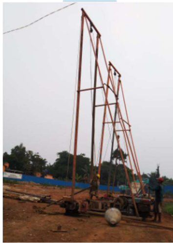
Gambar 3.8 Bored Pile Gawangan
