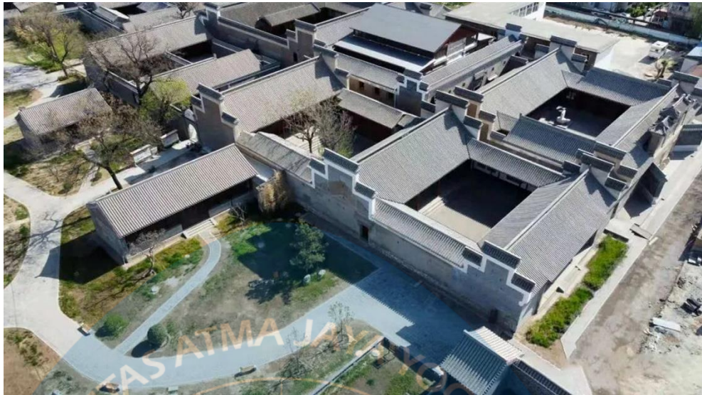
Figure 2.2 A Common Hui-Style Architecture Housing Complex with Multiple Courtyards
