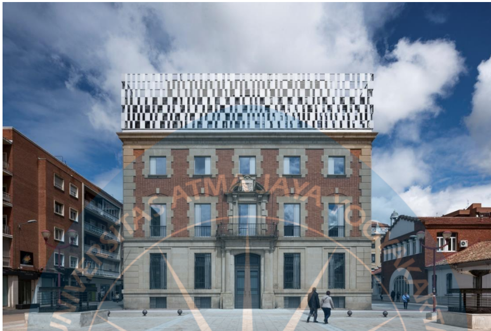
Gambar II.3. Refurbishment of the Justice Palace of Palencia (Sumber: archdaily.com)
