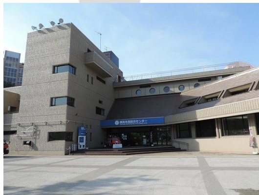
Gambar 2.5 Yokohama Disaster Risk Reduction Learning Center
