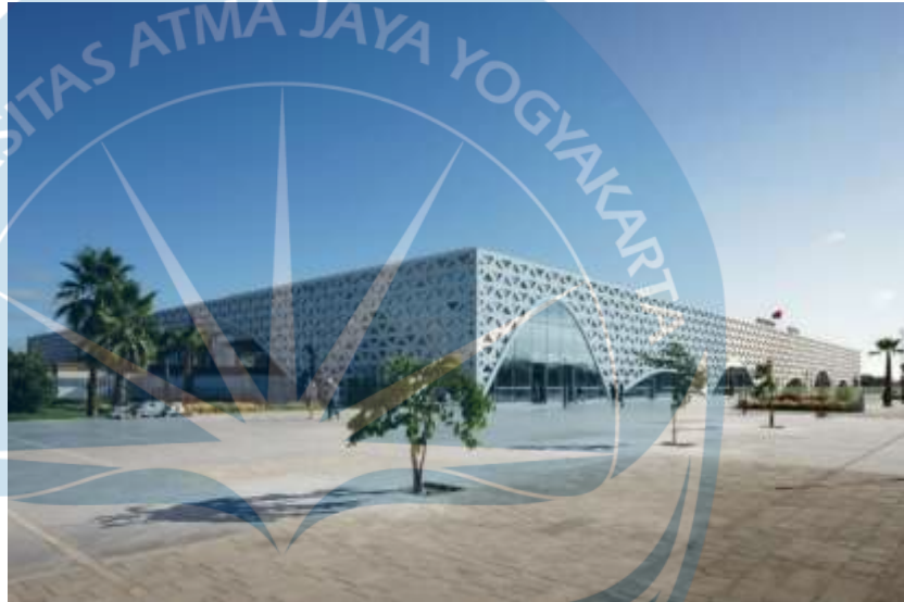
Gambar 2.1 Kenitra Rail Station
