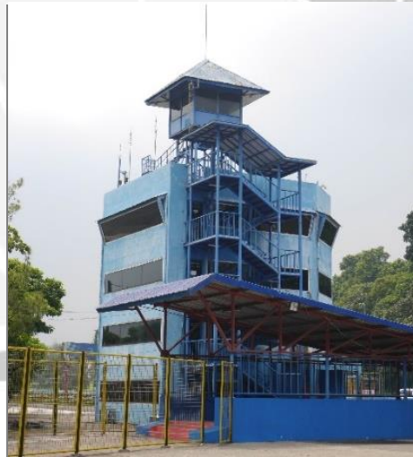
Gambar 2. 5 Race Control Tower
