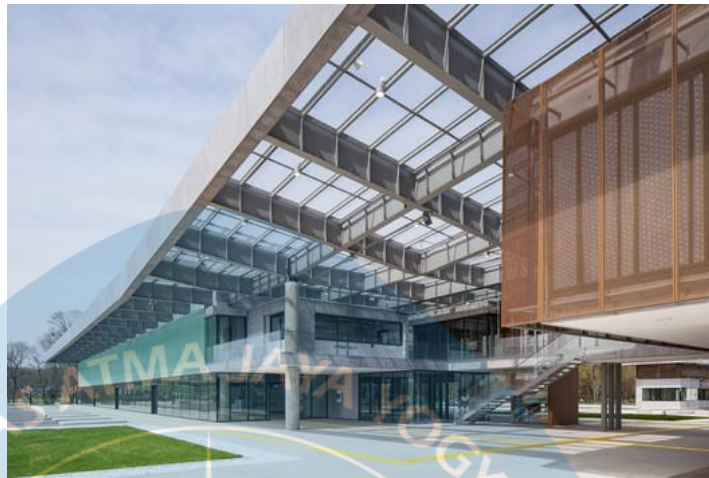
Gambar 2.9 Fasad Lüleburgaz Bus Station
