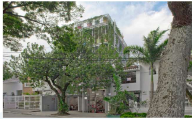
Gambar 2. 10 Fasad dari Bioclimatic Prototype of a Host and Nectar Garden Building Sumber https://www.archdaily.com/772039/bioclimatic-prototype-of-a-host-and-nectar-garden-building-husos
