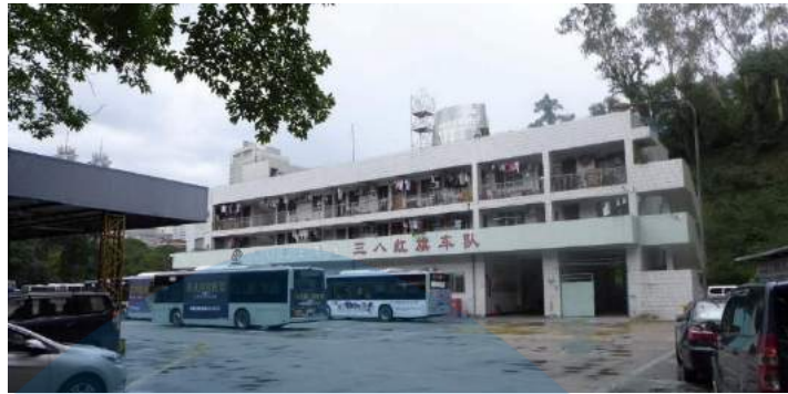
Gambar 2.27 Terminal Bus Lianhua Mountain Sebelum Renovasi Sumber : HAN , S., 2019. The Renovation of Lianhua Mountain Bus Terminal / CCDI - MOZHAO Studio. Archdaily.
