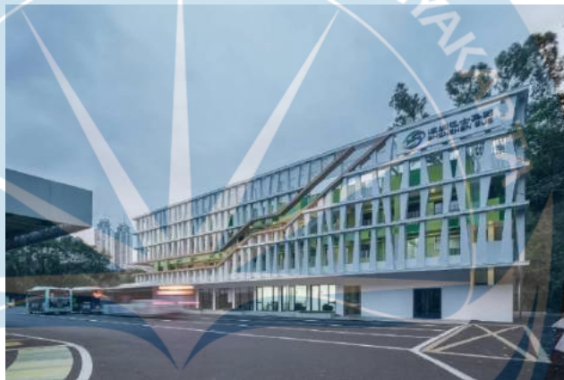
Gambar 2.28 Terminal Bus Lianhua Mountain Sesudah Renovasi Sumber : HAN , S., 2019. The Renovation of Lianhua Mountain Bus Terminal / CCDI - MOZHAO Studio. Archdaily.
