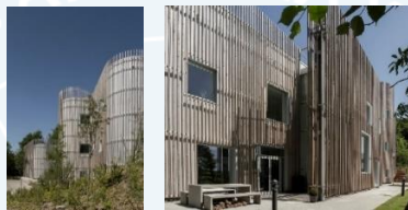
Gambar 2. 3. Fasad Livsrum Cancer Care Centre
