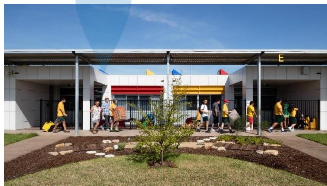
Gambar 2.7 Cairnsfoot Special Needs School
