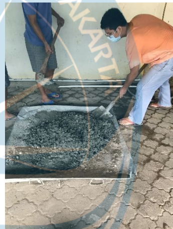
Mixing beton
